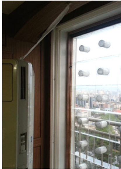
FIG. 7. An example of the air transparent soundproof window installed near a highway. The diameter of the air hole is 7cm. See Ref. 26.
